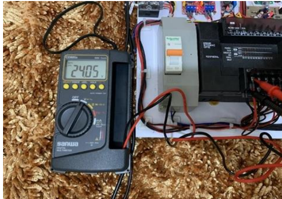
Figure 6. PLC Power Supply Voltage Measurement
